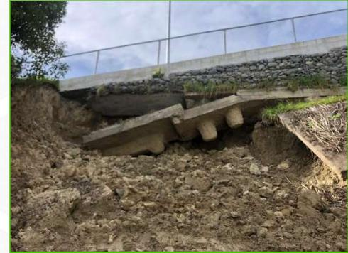
Abseil Access was approached to assist with the emergency support works for the Whaka Terrace roadway above the endangered house below at Enticott Place. The slip under the roadway was created by the saturation of the ground from a water feed under the roadway. We partnered with RDA consulting for the design of the temporary support works which are designed to be incorporated into the permanent solution. The works were deemed essential and conducted under Covid L3 restrictions.
