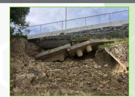
Abseil Access was approached to assist with the emergency support works for the Whaka Terrace roadway above the endangered house below at Enticott Place. The slip under the roadway was created by the saturation of the ground from a water feed under the roadway. We partnered with RDA consulting for the design of the temporary support works which are designed to be incorporated into the permanent solution. The works were deemed essential and conducted under Covid L3 restrictions.
