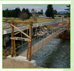
Main cable anchors and tower foundations are mass blocks 30mPa concrete. The 20mm IWRC main cables support 5 tons of deck as well as a 24kN live load. Abseil Access achieved deck stability using a unique continuously laminated kickboard and under deck catenary cables.
